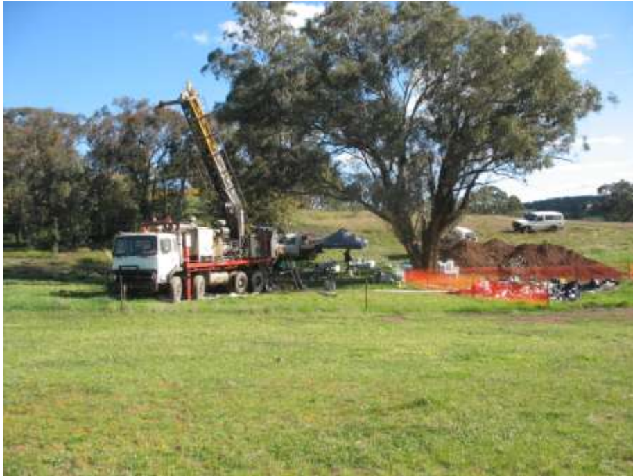
Figure 4: Copper Hill GCHR-314 in progress. See Figures 1, 2, & 3.
