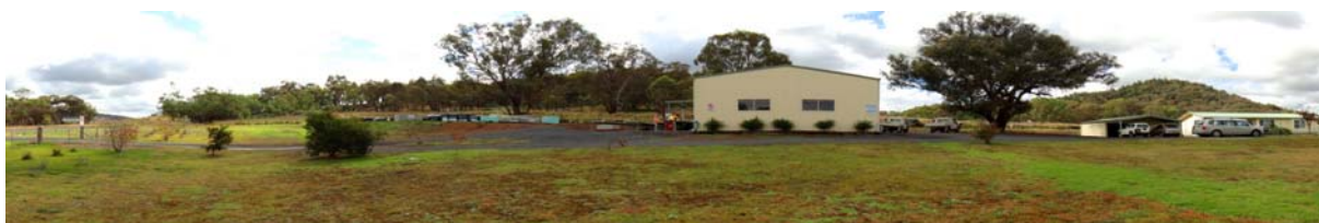
Panoramic view of 'Coppervale' - GCR's core shed, storage facility and site office for the Molong Project and Copper Hill, which rises in the background to the right-hand side of the picture. Photo: M. Alderdice
